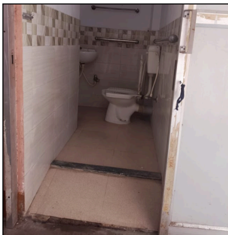
Entrance to wash room
